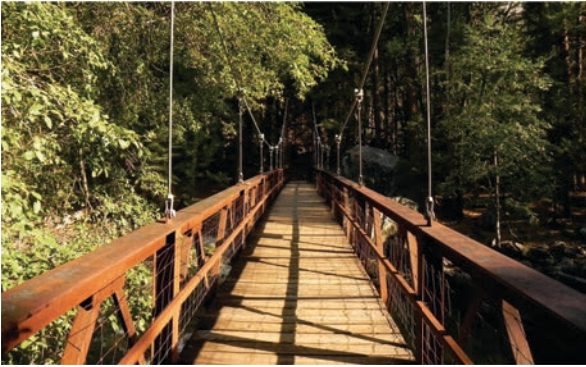
Kings River Bridge near Cedar Grove
